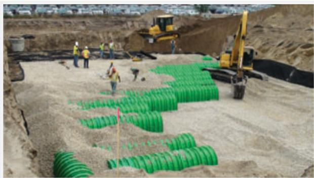
The site of the water retention system is backfilled up to six inches past the crown of the chambers.
