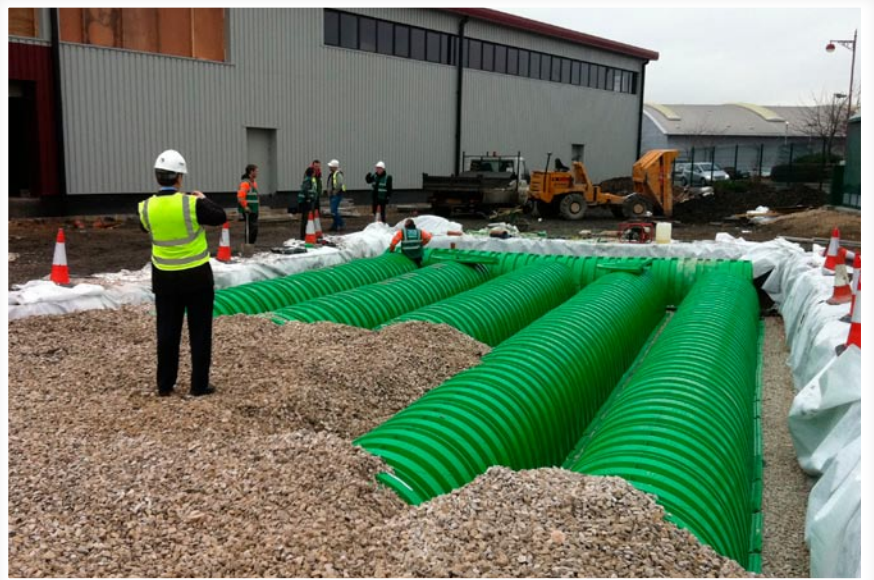
Triton SWS' innovative Main Header Row feeds five distribution rows in the Pride Park project.
