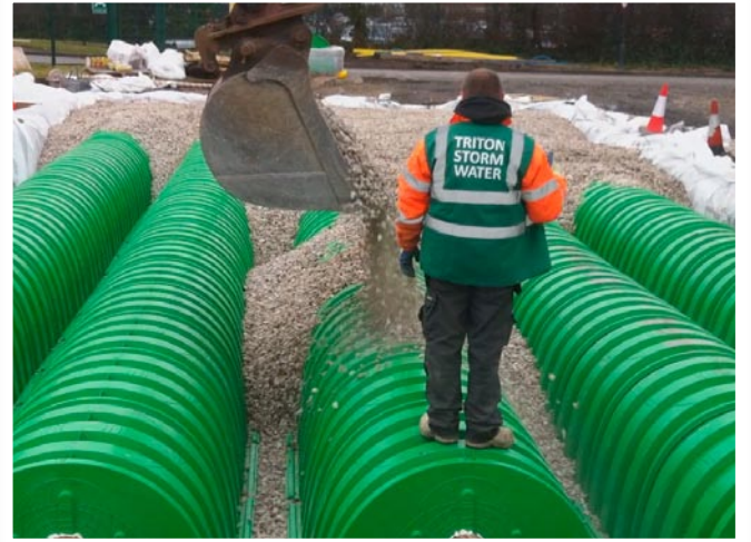
Triton SWS' impressive strength means that only 18" (457 mm) of backfill is needed before paving.
