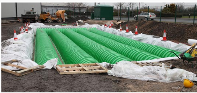
Small footprint; unrrialed storage. The Triton SWS system allowed stormwater storage for over 2,787 square meters of rooftop and a half-acre parking lot with just 114 chambers.
