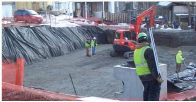
The Dubois project required a storage capacity of 11,500 cu ft of water, in a footprint that is 80' x 50'.
