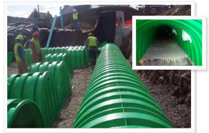
An integral Triton sediment catch basin (inset photo) was built into the Main Header Row.
