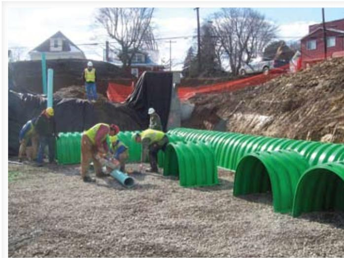
Lightweight and easy to handle, the Triton chambers can be placed without the aid of heavy equipment.
