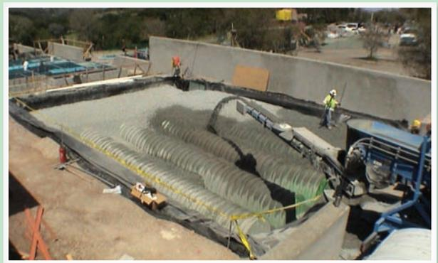
Less embedment stone backfill is required than with other systems.
