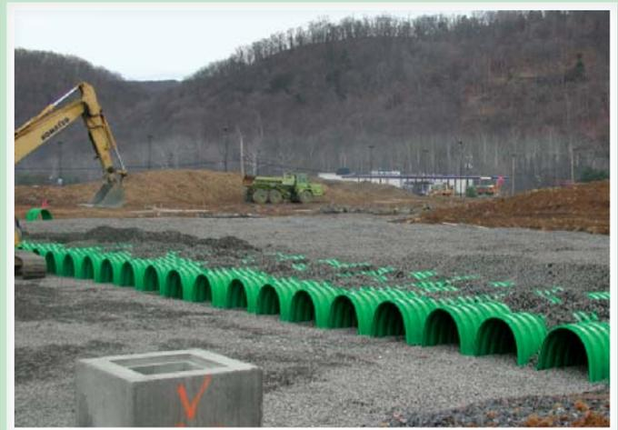
The enormous size of the site required the team to build and backfill in sections. The size of each section was limited to the reach of the excavation equipment. Because of the chambers strength, only 16" of cover was needed.
