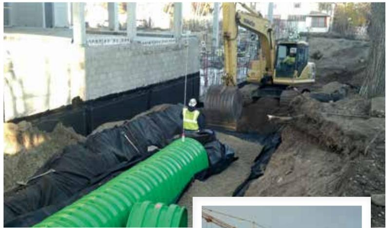
The strength of the Triton system was critical to the project. Developers were able to position the construction crane - weighing over 139,000 pounds with counterweights - over the installed chambers, saving them the trouble and expense of shutting down an adjacent street.
