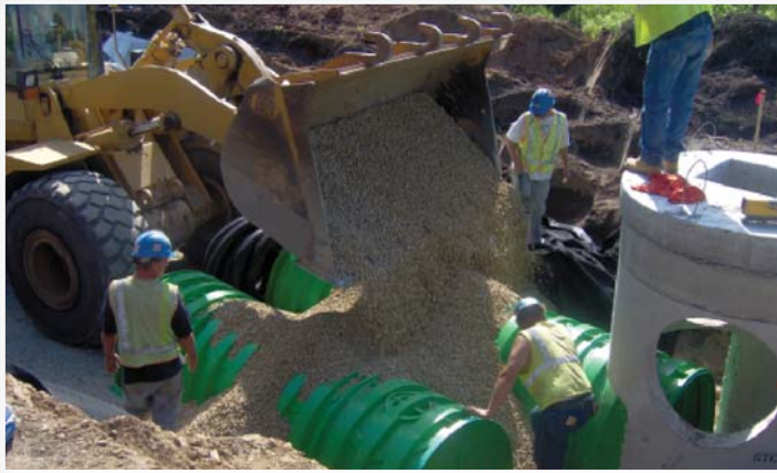
The site is backfilled with material to the determined elevation.
