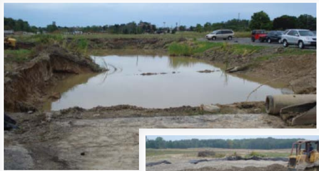
A detention pond was replaced with the Triton underground system allowing the dealership to add 60 additional parking spaces.
