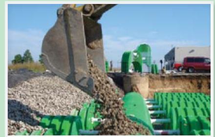
Backfill is added to the 33,000 cubic feet, Triton Stormwater Management System.
