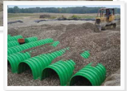
A detention pond was replaced with the Triton underground system allowing the dealership to add 60 additional parking spaces.
